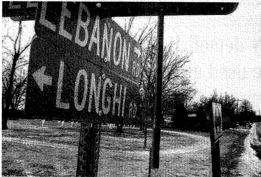
FILE PHOTO One of several 90-degree turns on Lebanon Road outside Collinsville. A plan to fix the twisty street has stalled.
